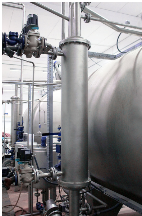
main heat exchanger along the machine
