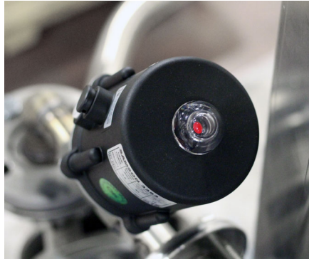
control valve for water
