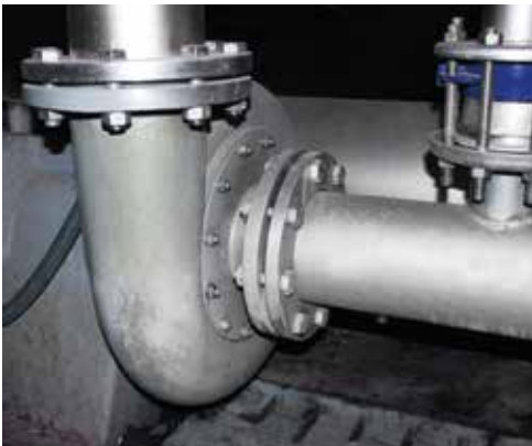
circulation pump 7.5hp for RAPIDDYE-150-1
