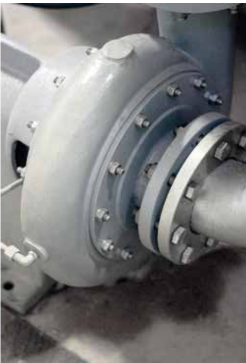
circulation pump 30hp for RAPIDDYE-100-7
