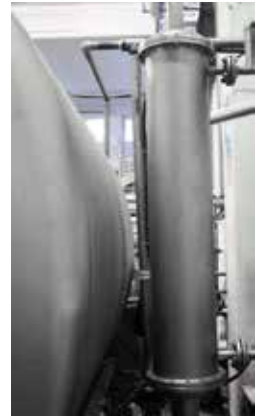
main heat exchanger
