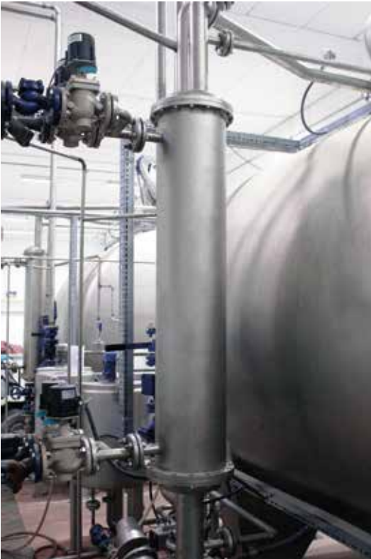
main heat exchanger along the machine
