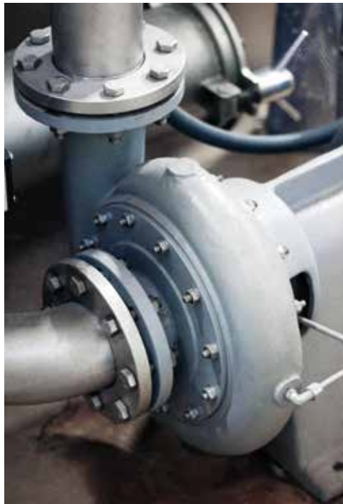
circulation pump 45hp for RAPIDDYE-150-8
