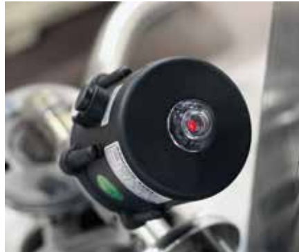
control valve for water
