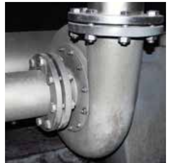
general view of circulation pump
